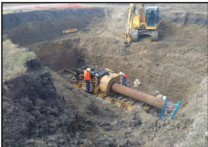
Pictured above: Installation of 18 inch Tee and 18 inch valve.
