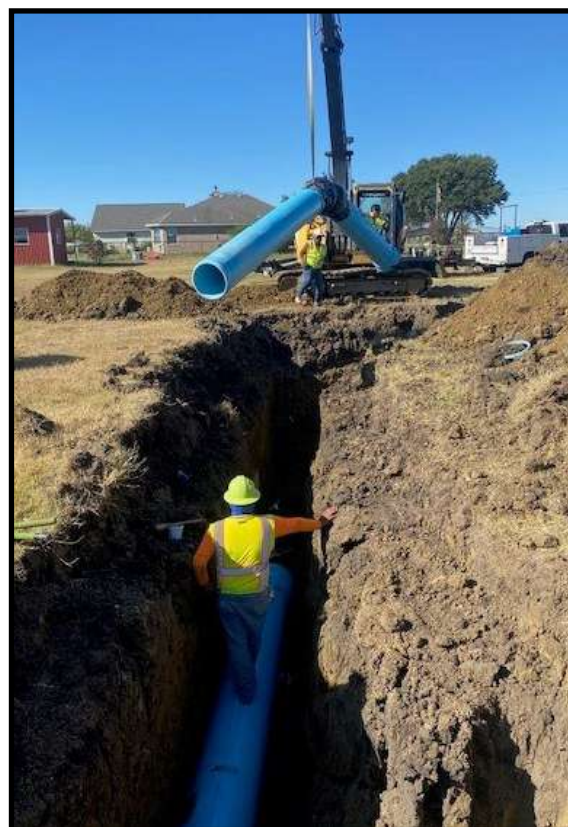
Pictured below: 45 degree angle of 18 inch pipe being installed.
