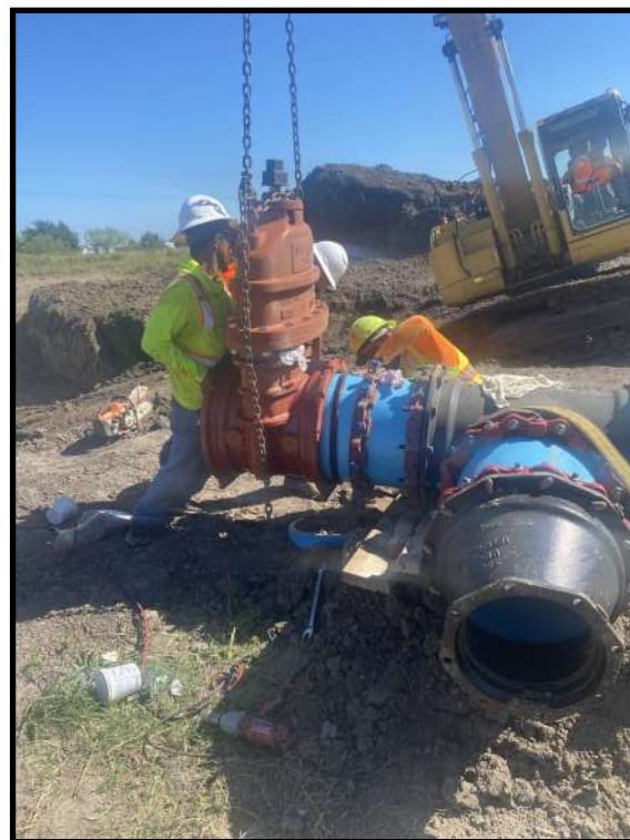
Pictured above: Installation of 18 inch Tee and 18 inch valve.
