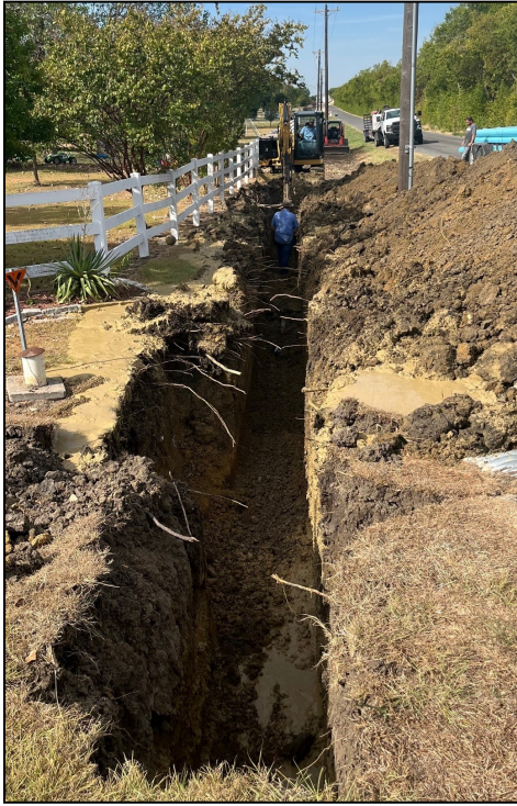
Picture on the Left: Installing the new 8" water line on Streetman Rd.
