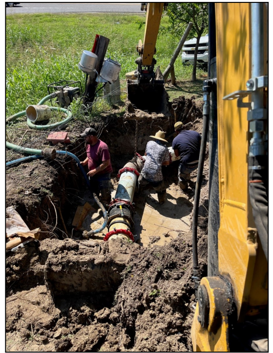
Picture on the Left: Installing the new 8" water line on Streetman Rd.
