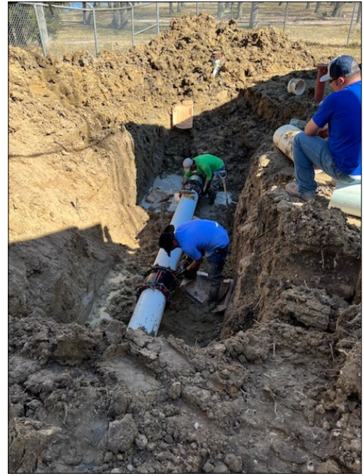
Pic 2: Repairing leak on 12" raw water line
