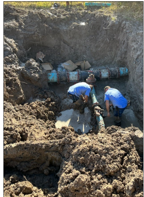
Pic 4: Repairing leak on 12" main
