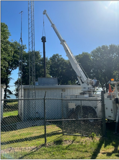
Pic 1: Pulling Raw Water Pump 2 for maintenance
