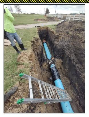
**Pictured to the left**: Performing a 32" road bore for installation of water line
